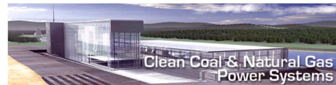
Clean Coal Power Plant Advanced Power Systems
