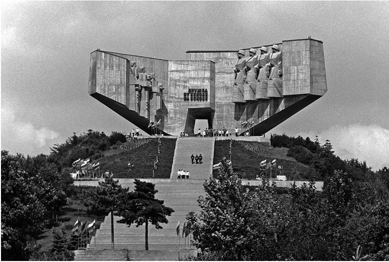
Figure 3. Park-monument of Bulgarian-Soviet Friendship in Varna. Source: Kafedjiiski et al. (1978). With the permission of State Archives, Varna.
