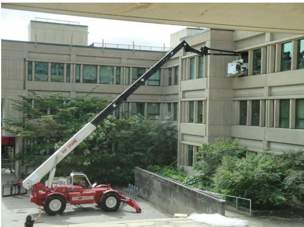
Delivery of the Nu ICP-MS required removal of a window. The unit was too large to fit in the elevator.
