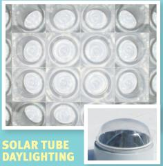
Solar tube skylights pull a dramatic amount of "ducted daylight" into the second floor open office space producing up to 20,500 lumens each. In this regularly occupied space, the solar tubes minimize the need for artificial lighting during normal daytime occupancy.
